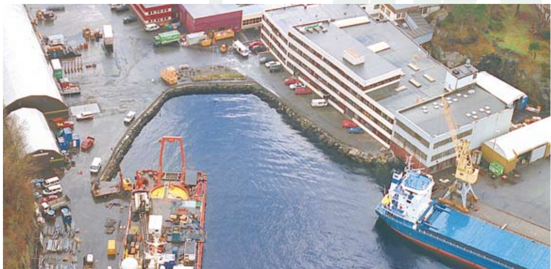
W. Giertsen Services AS's quay and warehouse at Nygårdsviken in Bergen, Norway.
